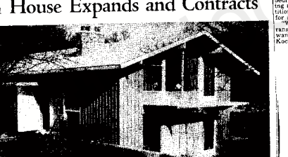
THE "ATTIC AND BASEMENT" HOUSE—Model home in Weston which has two stories, but looks like a ranch house. It has four feet underground, lower floor is down one-half flight of interior stairs, and top floor is up one-half flight. Gable ends are largely glass.
