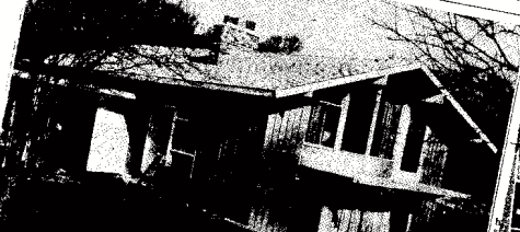
The house that "Tech Built" in Weston, Mass., is for the growing family. Rooms can be moved upstairs or downstairs, and changed in size according to the fluctuating needs of the owners.
